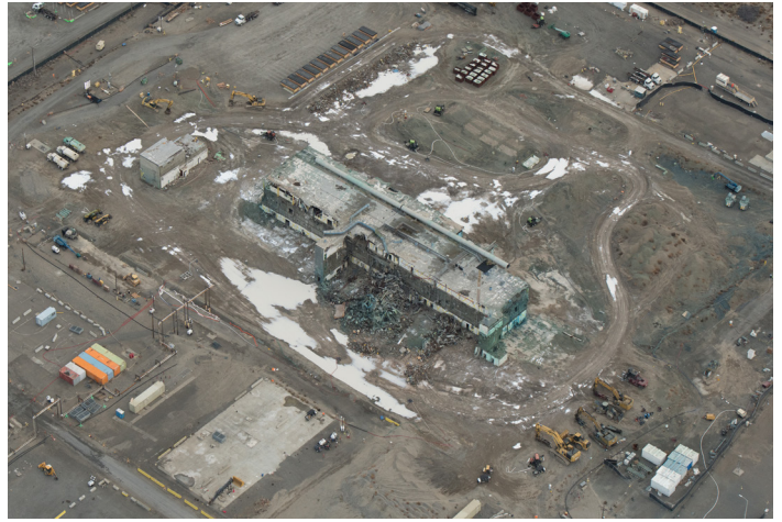
The skyline at the Hanford Site changed for the better as workers safely leveled the main processing facility at PFP.
