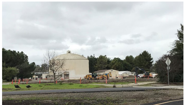
LLNL Building 280 Area - March 2019.
