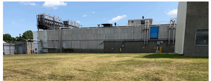
Restored area where Building G2 stood.
