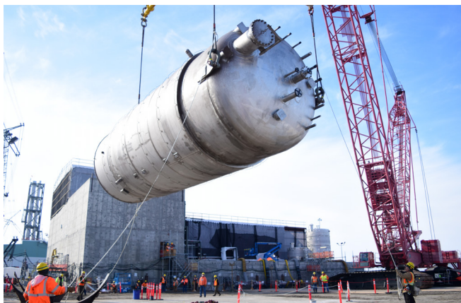
The entire site is supporting a shift to 24/7 operations to treat tank waste, including workers building the Effluent Management Facility for treating secondary waste from vitrification.
